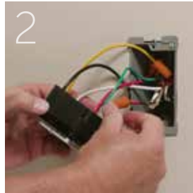
Remove existing switch
