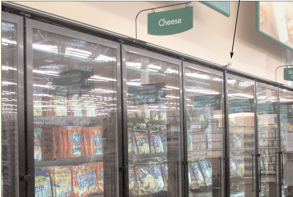
Williams explained that fluorescent lighting in refrigerated cases is very high maintenance due to condensation and resulting corrosion of contacts in the lamp holders. To maximize energy savings and LED life, the time delay for the sensors was set to the minimum of 30 seconds.
