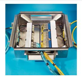
Enclosure for 6" deep floor. Two pairs of pivoting mounting rails for 19" patch panels. Rails support 2 RMU each.
