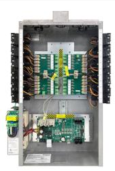
The LMCP series panels are available for Dimming (LMCPx-10V) or Switched(LMCPx) control of lighting and plug loads. The panels can be networked together to enable automation through out an entire facility. The HDR panel relays respond to inputs from Digital Lighting Management (DLM)
